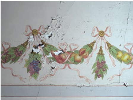
Fig. 1: Flaking area on the north side of the ceiling before intervention (in raking light).
