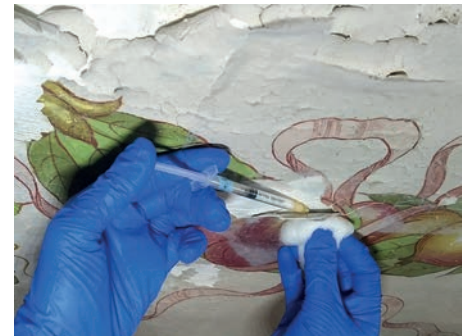
Fig. 3: Injection of adhesive behind a large lifted paint flake.
