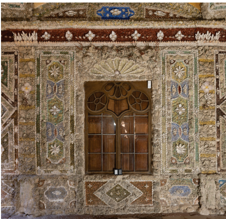
Fig. 1: St Mary Magdalene Hermitage, north wall of the chapel, tufa fragments, pebbles and shells are designing the baroque pattern. The pebble areas are elaborately decorated with multiple paint layers including the application of glass and metal particles.
